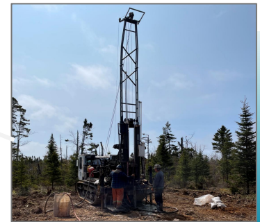
Geotech work for MET
