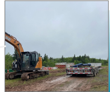
Met towers installed
